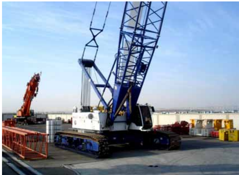
KN's first crawler crane, a Liebherr Model-LR 1160
